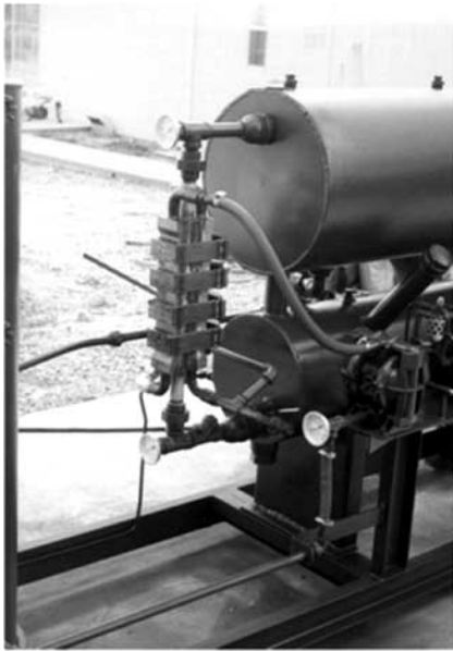
Fig. (16). Photograph of a thermoelectric power generator produced power for cathodic protection of the well and gas line, which used the temperature difference between hot and cold legs of glycol natural gas dehydrator cycle [15].
