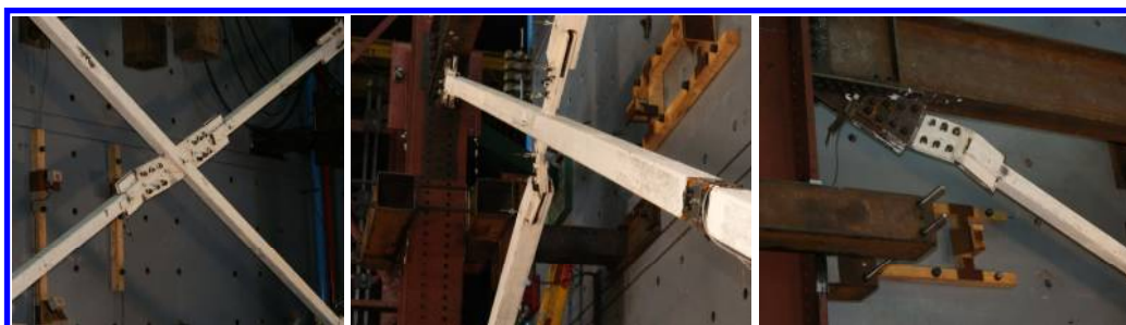
Figure 2. Connection instability observed in the tested specimens.
