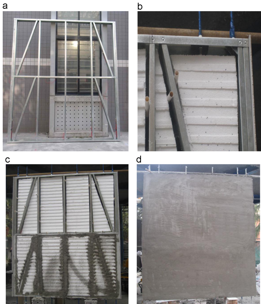
Fig. 7. Construction procedure of wall specimens with SLM on both sides: (a) assembling of the CFS members, (b) installation of the EPS boards, (c) covering of the CFS members with mortar, and (d) spraying of lightweight mortar on both sides.
